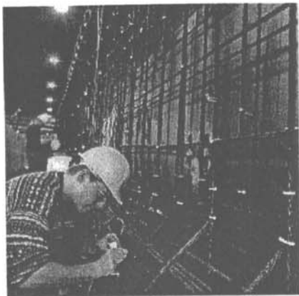
Figure 2.16 The installation of FBG sensors along pre-stressed girders (left). The Taylor bridge is being monitored by the FBG sensors (right).
