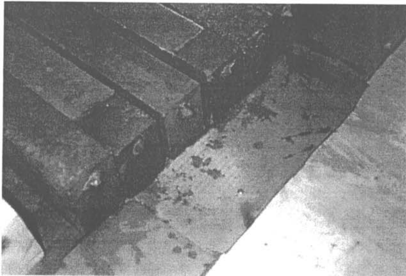
Figure 7.3 Both ends of the embedded steel bar are protected by rubber element.
