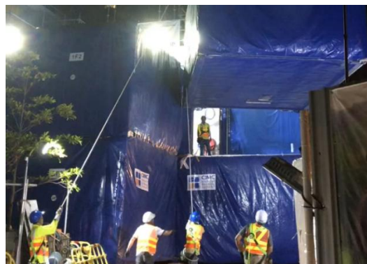
Figure 4-4 On-site MiC Lifting Placing Movement (Stage 5)
