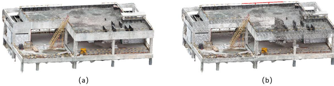
Figure 29 The detected result of the missing guardrail: (a) standard point cloud of simulated scenery 1 and (b) detected results of the missing guardrails in scenery.
