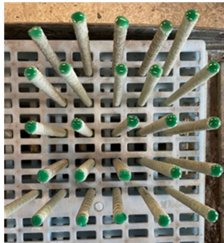
Figure 5.2. Sealing of bare bars
