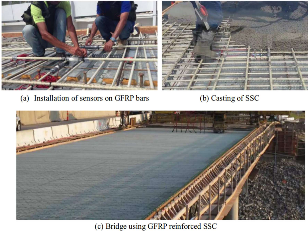
Figure 1.3. Demonstration project of GFRP reinforced seawater sea sand concrete structures (Xiao et al. 2017)
