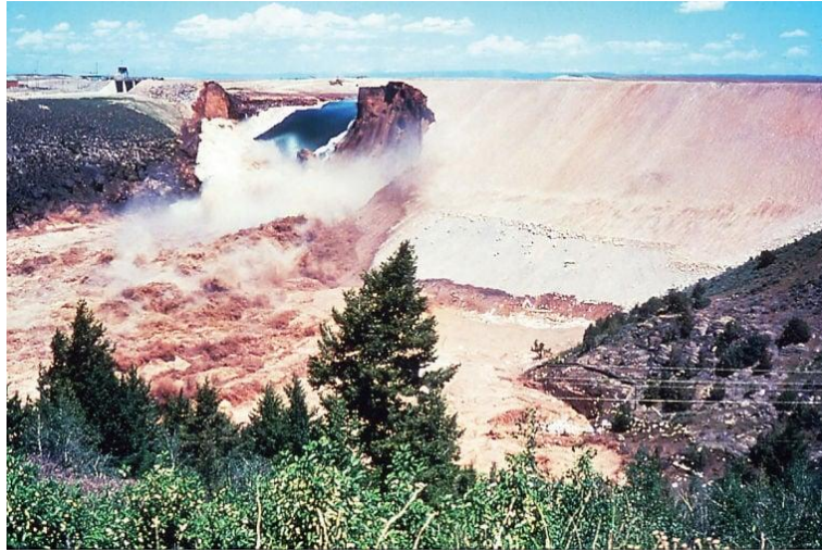
Fig 1.1 Failure of the Teton Dam due to internal erosion in Idaho, USA, in 1976 (USBR 1976).
