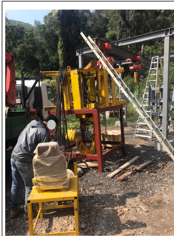
Figure 4.12a: Record Photo of Installation
