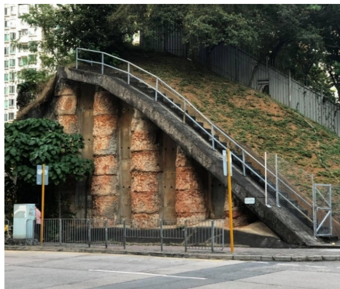
Figure 1.1: Earth Retaining Structures by Caissons
