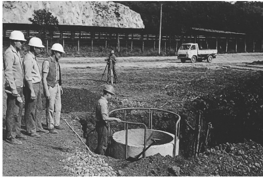
Figure 1.2a: Starting of a Caisson (Law 1981)(redrawn)
