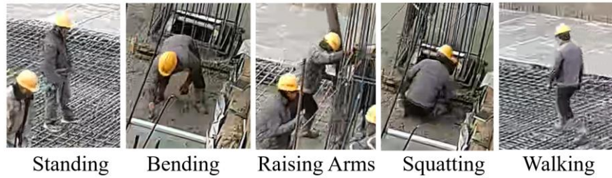
Figure 4.10 The postures considered in the concrete pouring case
