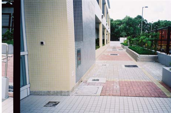
Figure 2.5.1 Recycled paving blocks in Yuen Long [Poon, 2004b]
