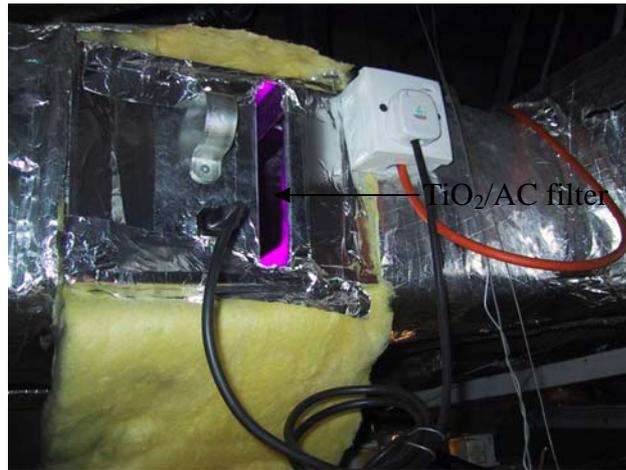
*Fig. 3.8* TiO<sub>2</sub>/AC filter installed in an air duct.
