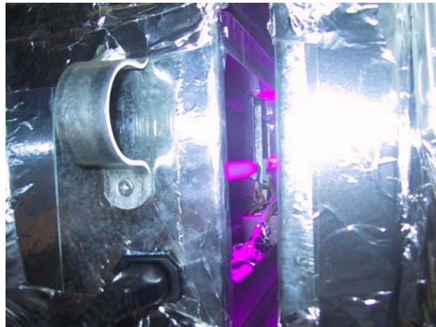
*Fig. 3.9* UV lamps installed inside the air duct.
