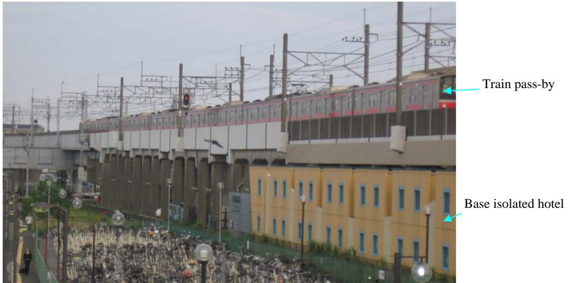
Figure 6.6. Photograph of a train pass over the isolated box (hotel) in Japan (Tokyo)
