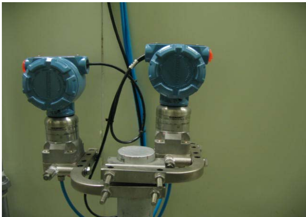
Photo 10 Manometers for measuring supply air static pressure
