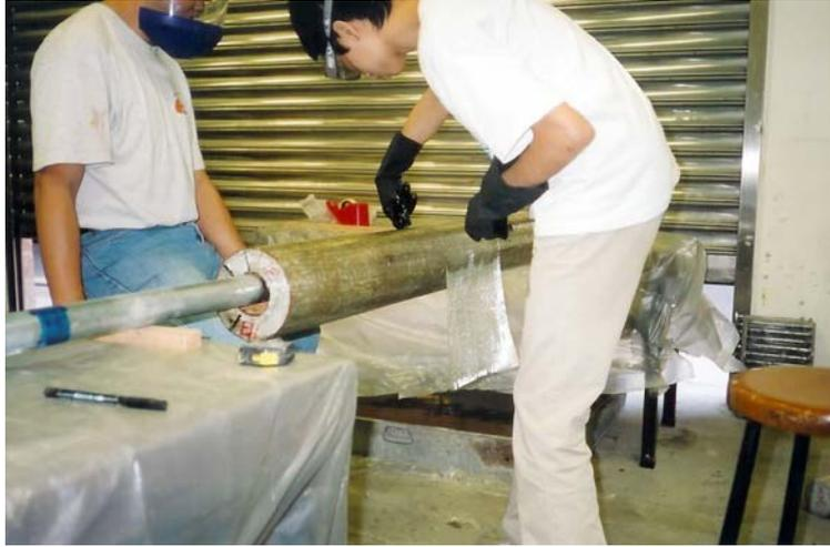
Figure 6.5 Fabrication of FRP tube
