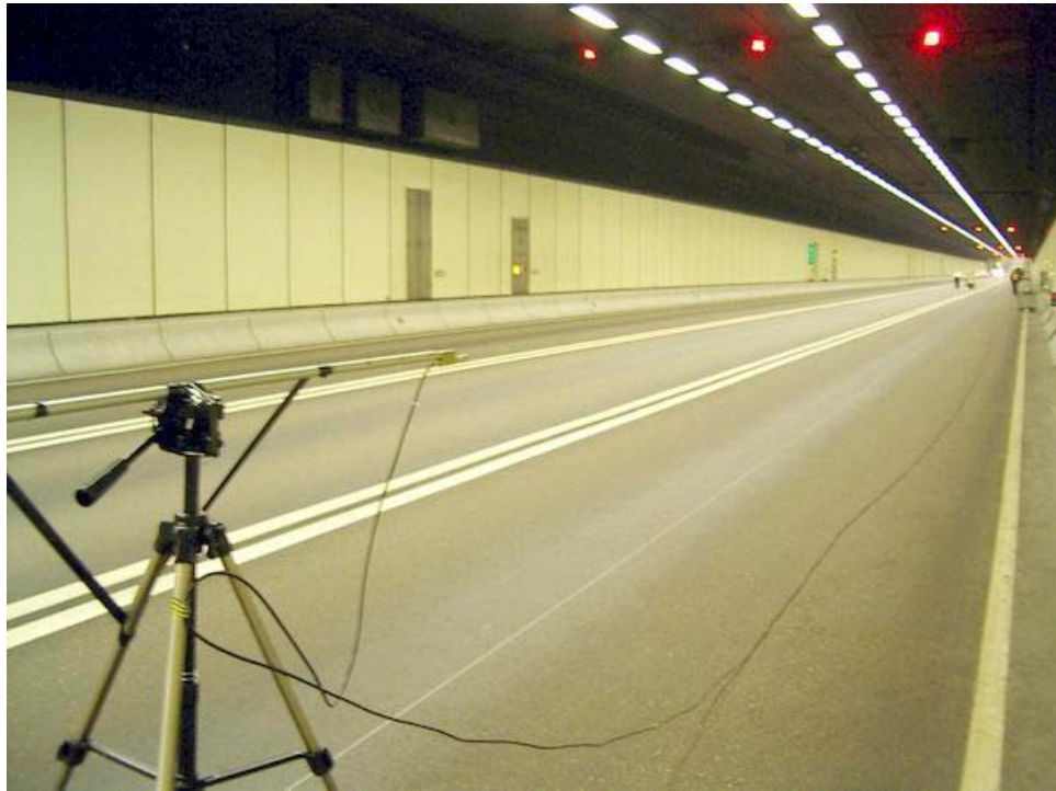
FIG. 2.6: The Western Harbour Tunnel.
