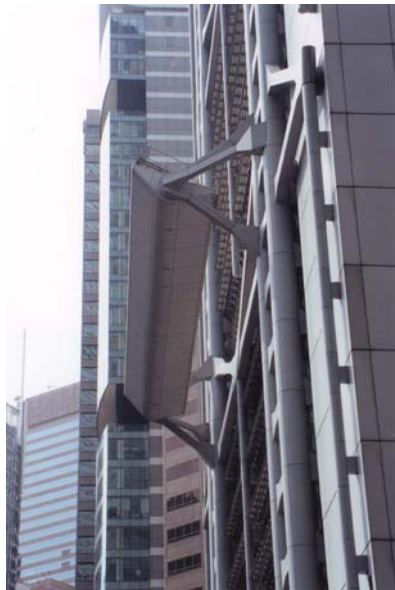
(c) "Sunscoop" device (directing sunlight into the atrium)
