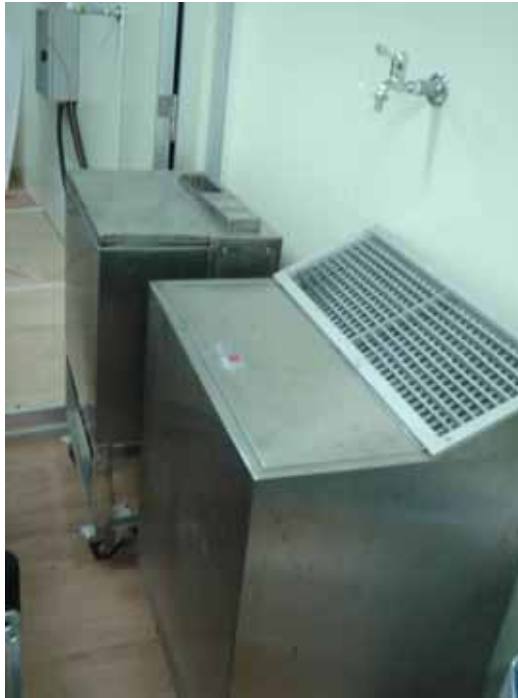
Photo 5 Load generation units inside conditioned space
