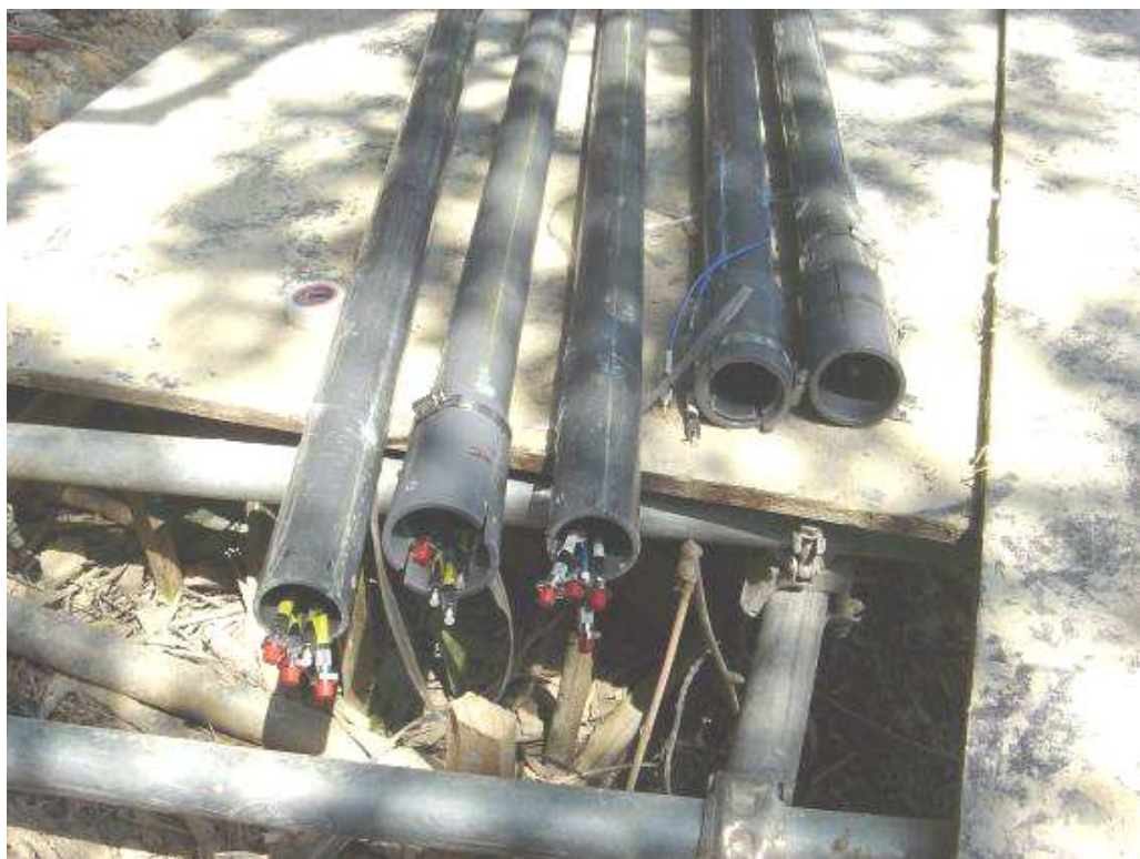
(a) Details of the FBG inclinometer prior to installation
