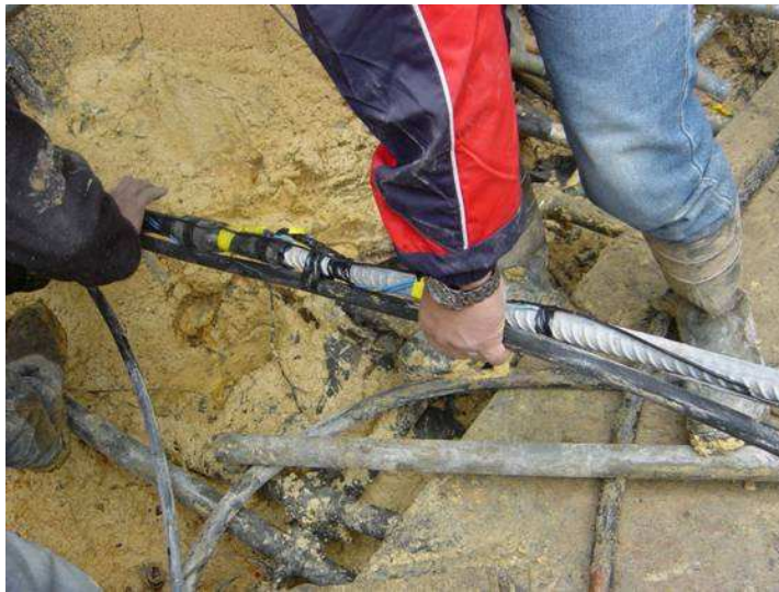
(c) Connecting optical fiber cables at the coupling part
