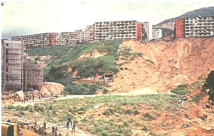
Figure 2.2 Sau Mau Ping Landslide (1972)
