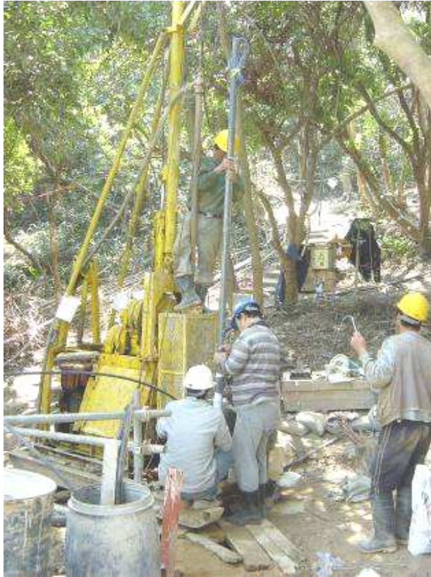
(b) Inserting of the FBG inclinometer in the drillhole
