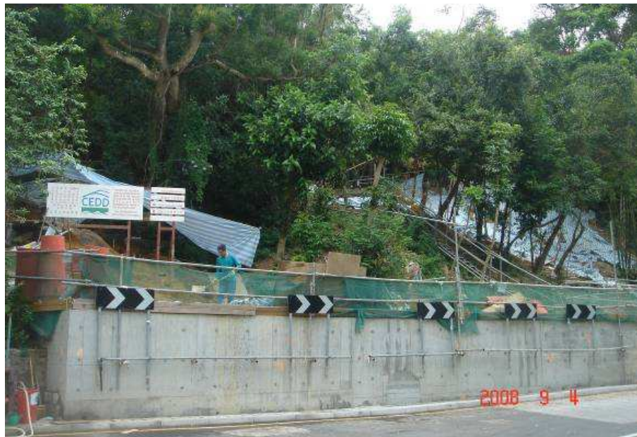
(e) Constructed soldier-pile retaining wall
