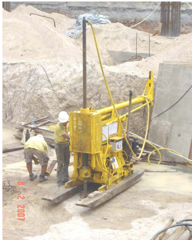
(a) Preparation of a borehole for installing the FBG settlement tubes
