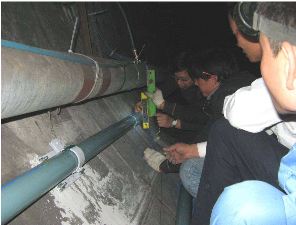
Figure 3.33 Installation of the FBG in-place inclinometers in Shanghai Metro No. 2 for displacement measurements
