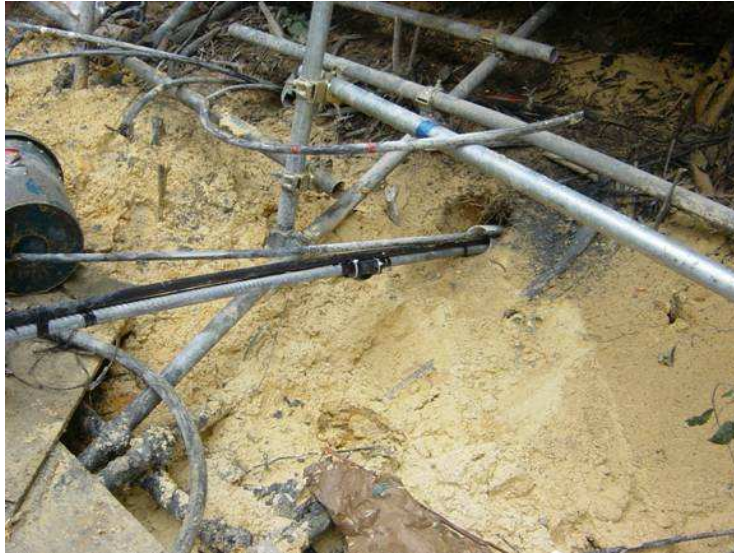
(b) Inserting the soil nail in the drillhole
