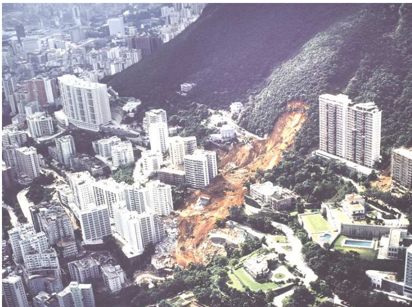
Figure 2.3 Po Shan Road landslide (1972)
