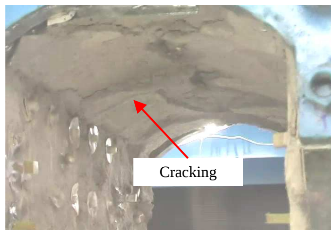
(b) Crown of the power house under an overburden depth of 1400 m
