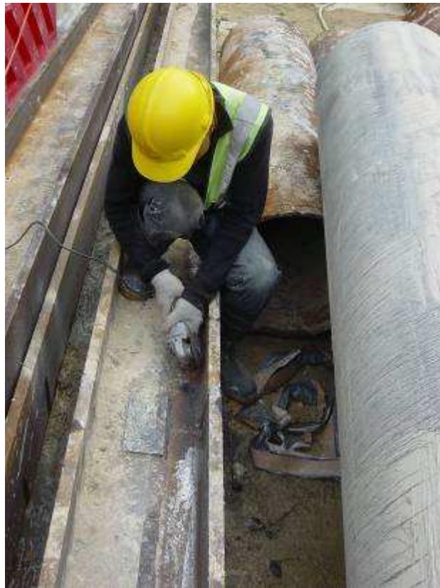
(a) Polishing of the H-shaped steel
