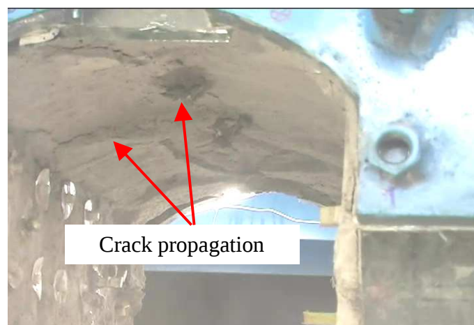
(c) Crown of the power house under an overburden depth of 1600 m
