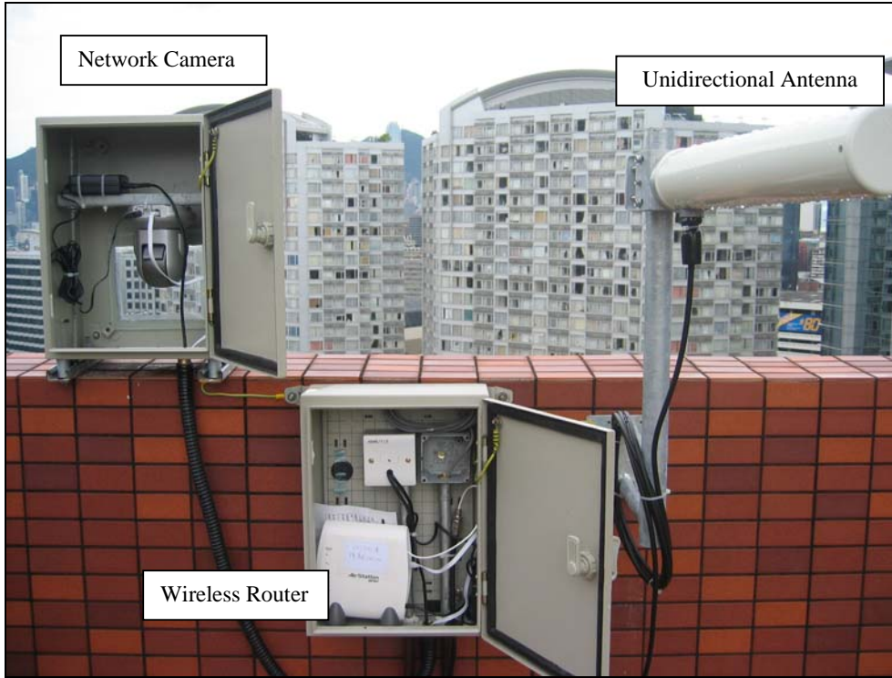
Figure 18. Installation setting of the monitoring viewpoint (Site A)
