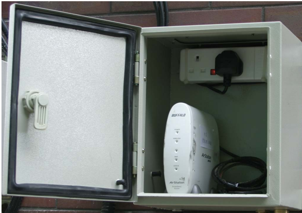
Figure 11. Metal cabinet with rubber weatherproof sealing
