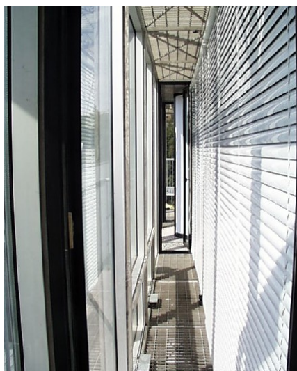
Figure A-8: Multi-storey naturally ventilated double façade
