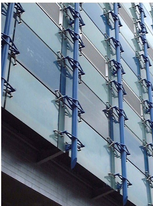
Figure A-10: Exterior of the double skin façade
