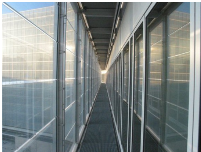
Figure A-7: View of the large cavity and the louvers in vertical position
