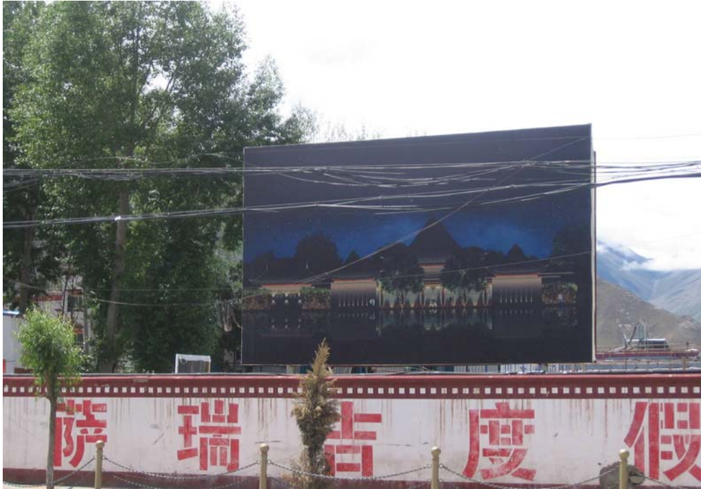
Photo 4-11: Construction site of the St. Regis Hotel, Lhasa
