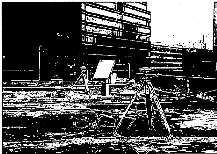
Figure 5.3 Experiment set up at the roof top of the HKPU
