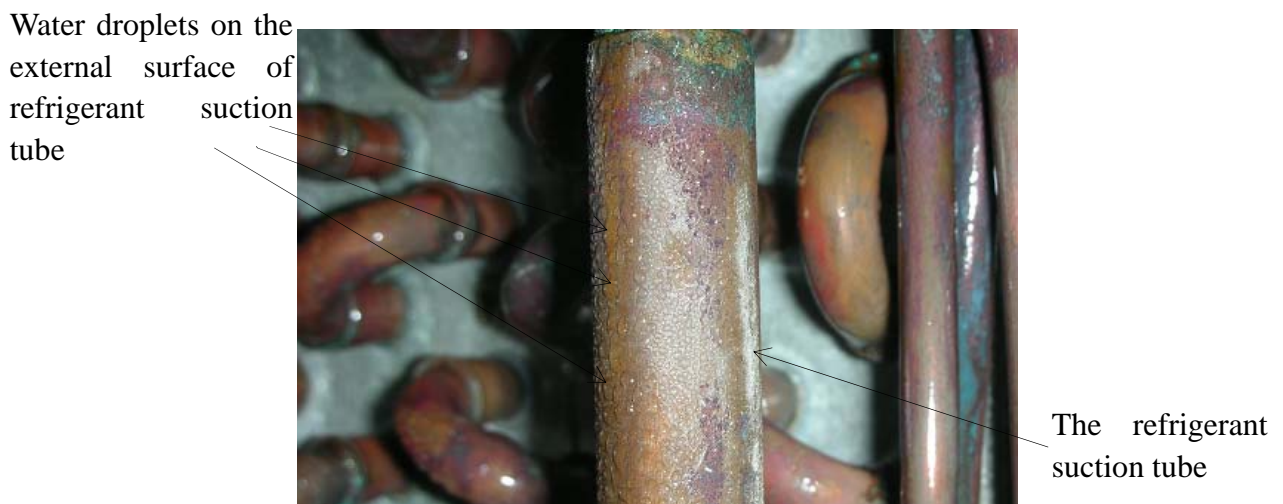
Fig. 6.1 Water droplets formed on the surface of a refrigerant suction pipe
