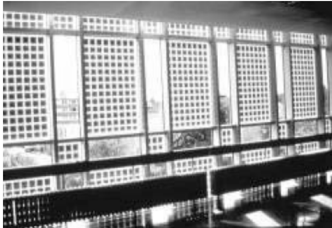
Figure 2.1 Example of a semi-transparent PV façade
