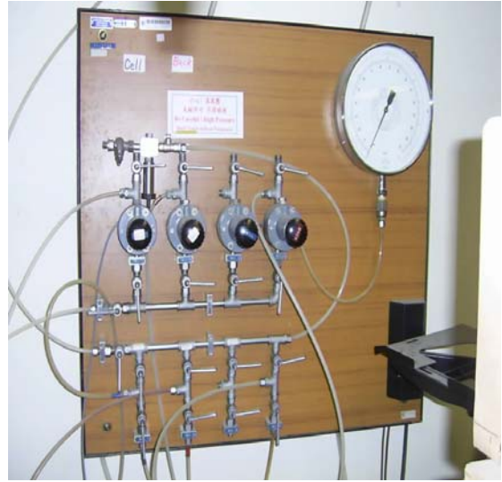
(b) air and water pressure regulator panel
