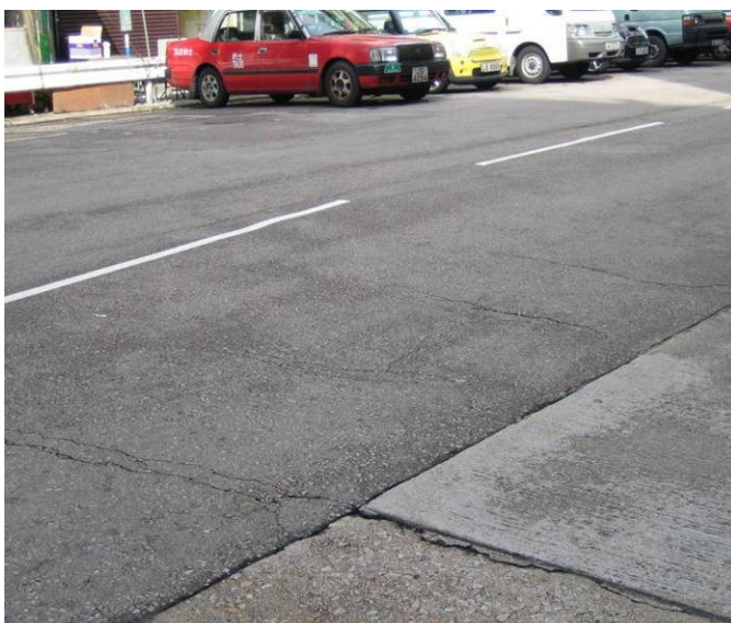
Figure 2.18 Block Crack
