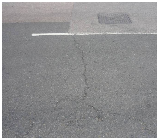
Figure 2.23 Transverse Crack
