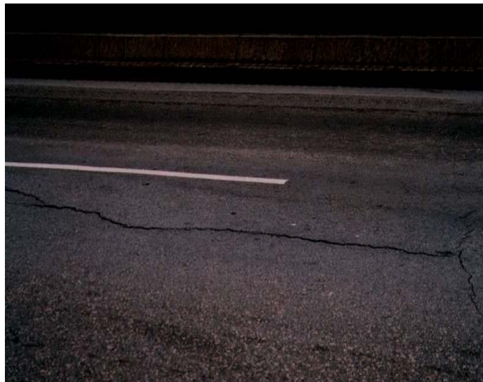
Figure 2.21 Longitudinal Crack
