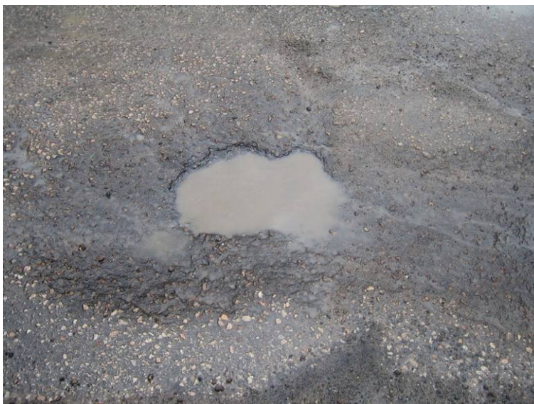
Figure 2.31 Pothole
