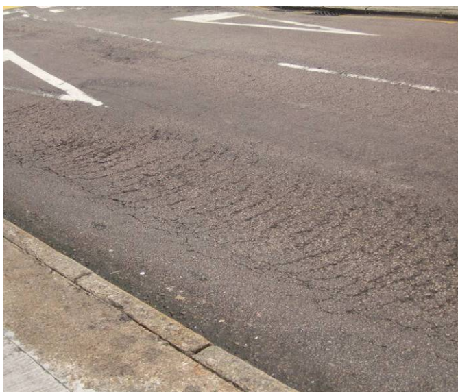
Figure 2.22 Slippage Crack
