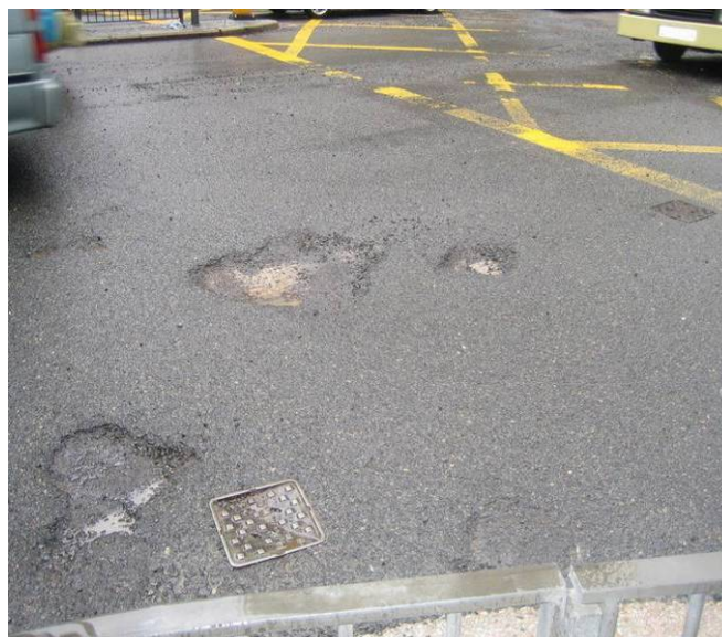
Figure 2.32 Delamination
