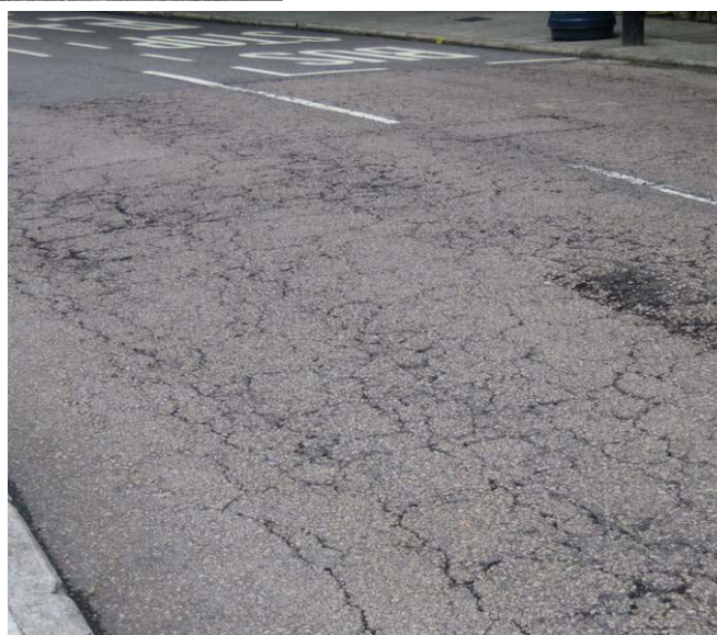
Figure 2.19 Crocodile Crack
