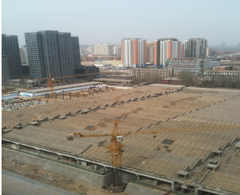
Zigzag factories surrounded with construction sites and high rising buildings
