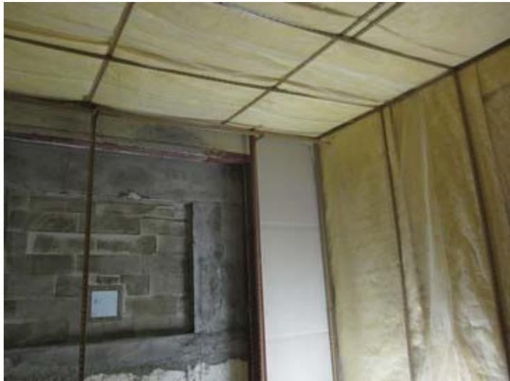
**Figure A.4 A view of one of the two chambers after plate installation**
