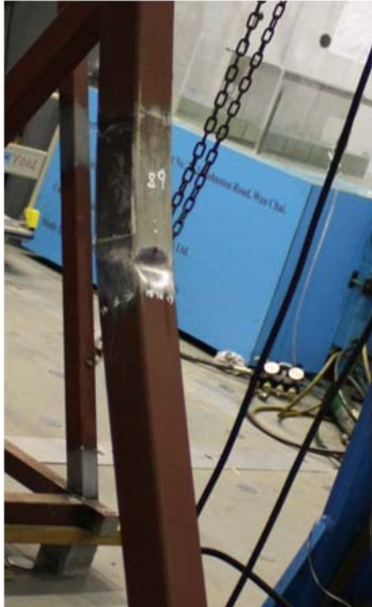
Inward buckling in steel tubular member
