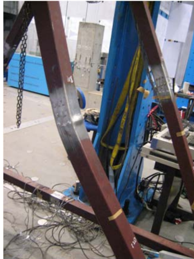
Outward buckling in CFS tubular member
