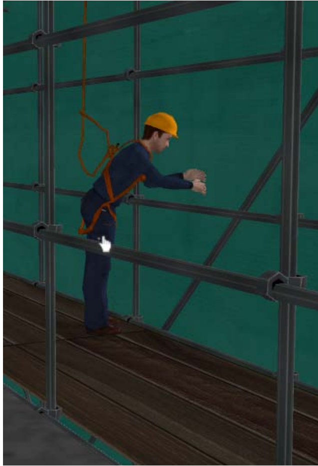
Figure 5.9. Working at height without safety belt
