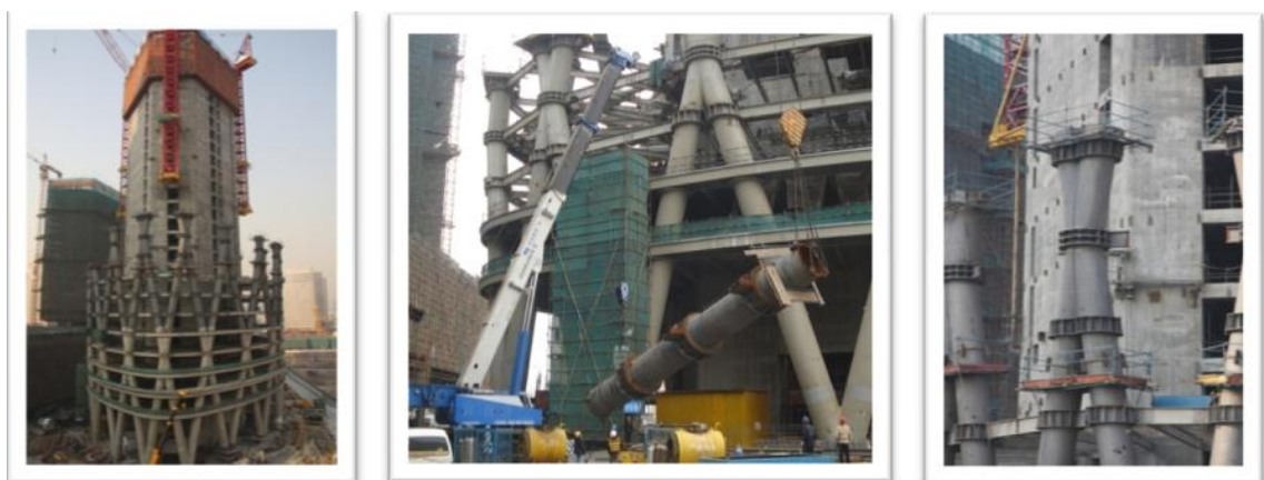
Figure 1-1: The real case of large-scale structural steel components assembly
