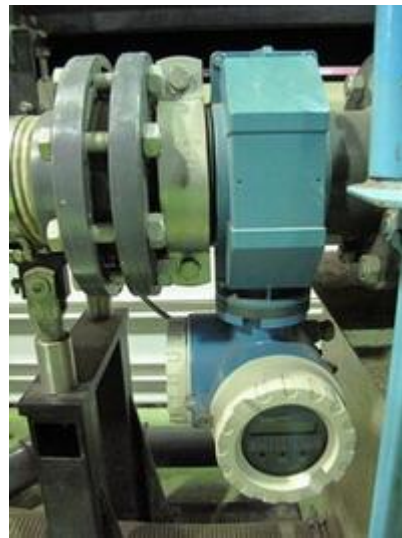
Photo 5.2. The build-in electromagnetic flow meter
