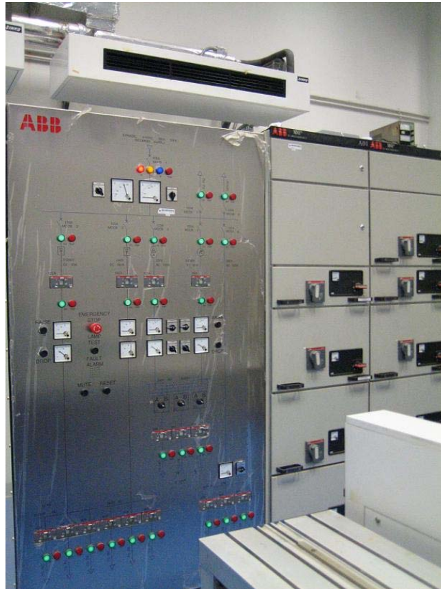
Fig. 6.6 The 400 V, 1,000 A, 3-phase electrical switchgear made by ABB Xiamen Low Voltage Equipment Co. Ltd. and installed in the Electrical Machines Laboratory (EF001a) of the Department of Electrical Engineering at PolyU.
