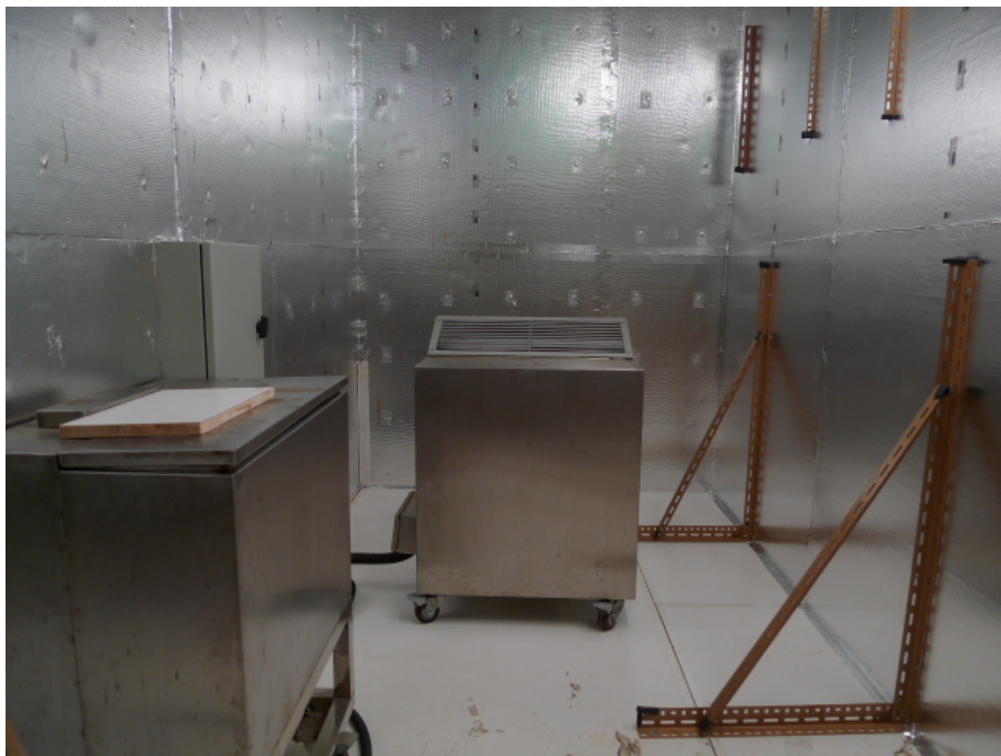
Photo 4 Load generation unit inside conditioned space
