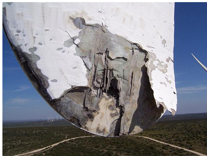
Figure 1 Wind turbine blade destroyed by a lightning strike
