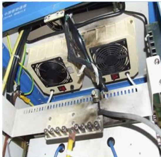
Figure 2 Damaged telecommunication device in the radio base station.
