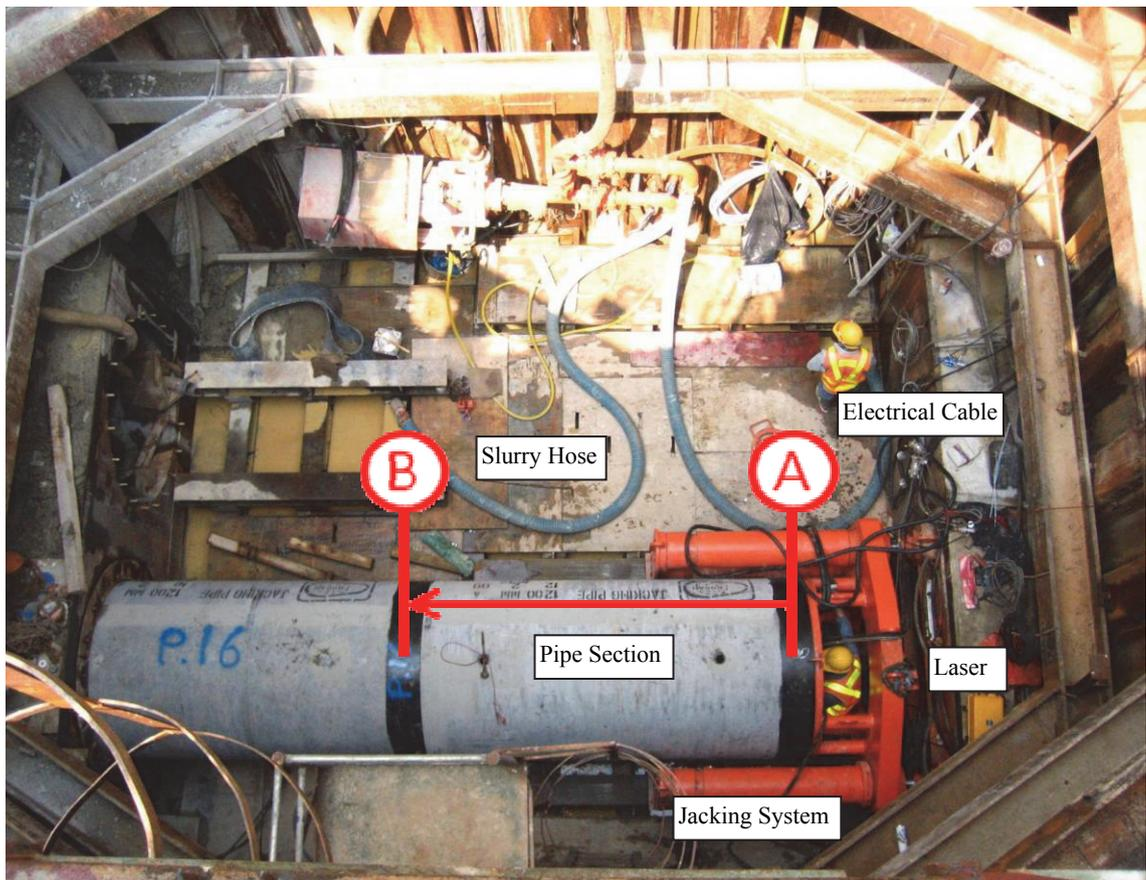
Figure 5.6. Jacking Pit Layout of So Kwun Wat Microtunneling Project
