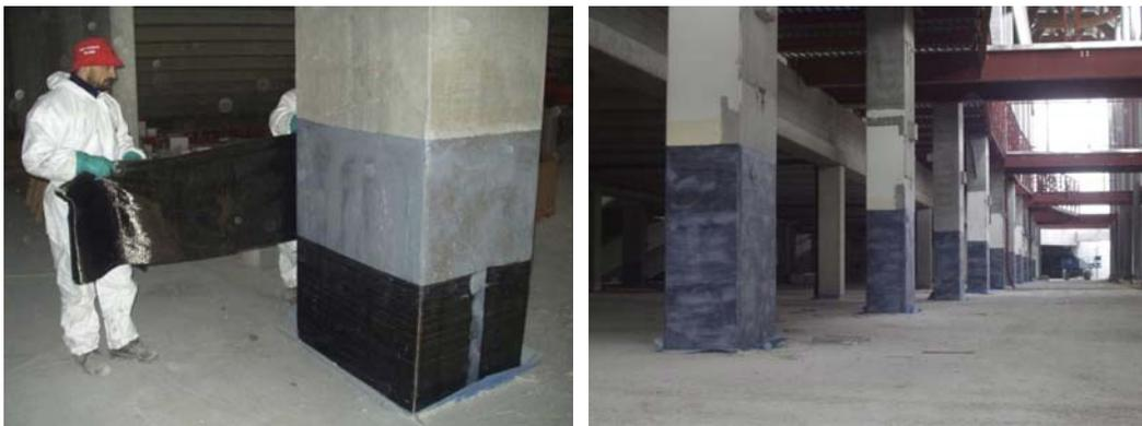
Figure 2.2: Seismic retrofitting of concrete columns
