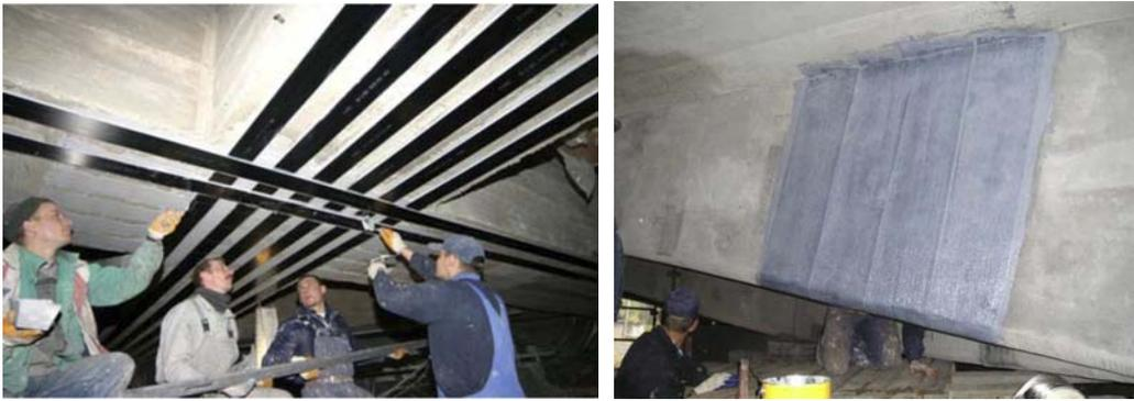
Figure 2.1: Flexural and shear strengthening of concrete beams
