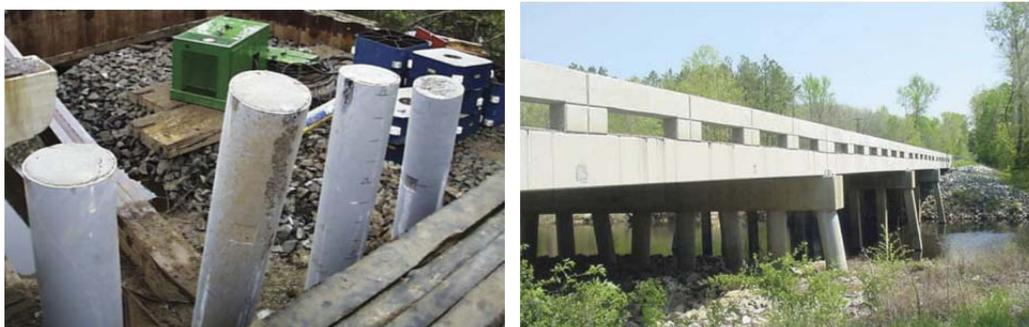
Figure 2.6: FRP tubes in new construction (Fam *et al.* 2003)
