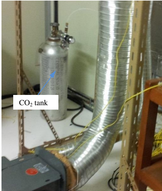
Photo 6 The CO 2 tank
