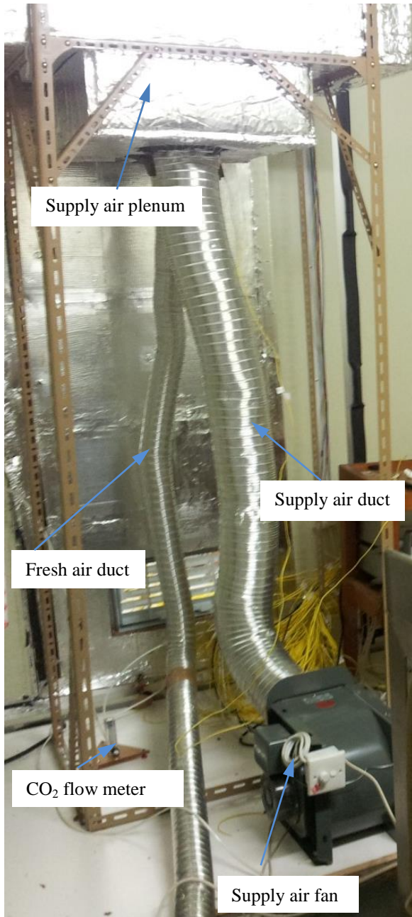
Photo 4 Supply air plenum and flexible ducts
