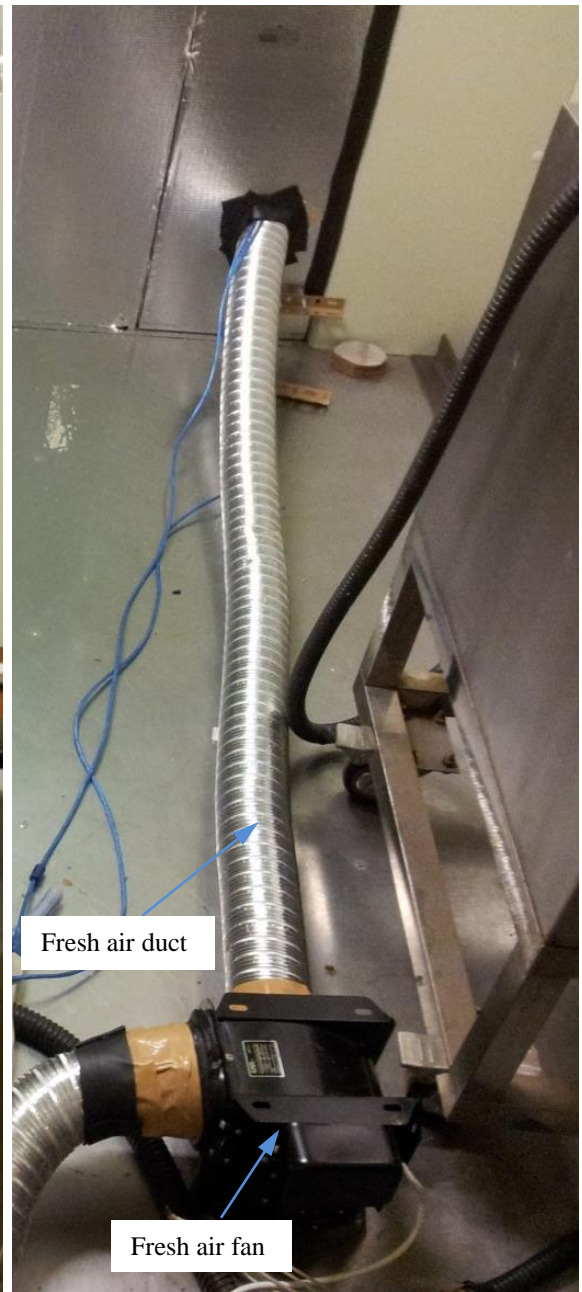
Photo 5 Fresh air duct
