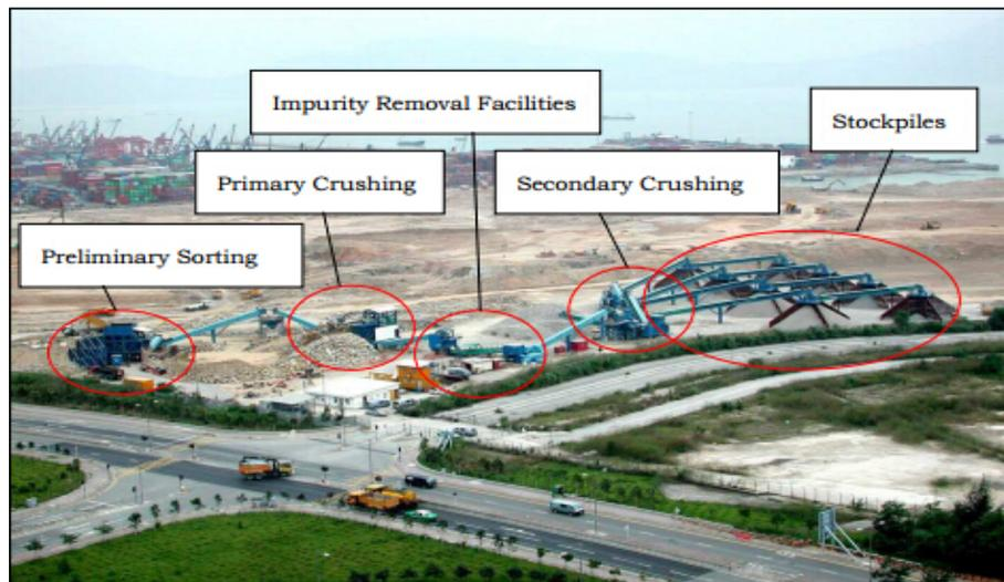
**Figure 2-2 -Pilot C & D Material Recycling Facility in Tuen Mun Area 38 (EDB 2011)**
