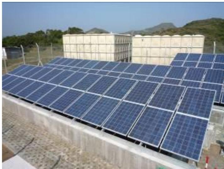
Fig. 8.1 The installed PV system on a remote island in Hong Kong (19.8kWp)
