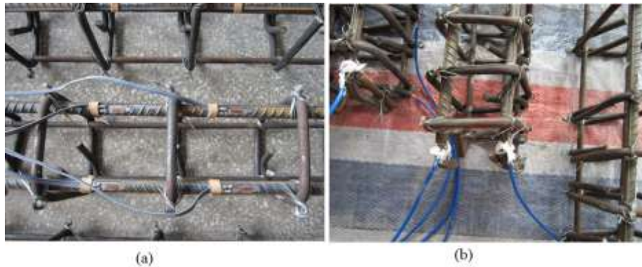
Figure 4-2 Measurement of tensile steel reinforcement (a) strain gauges; (b) lead wires for corrosion monitoring
