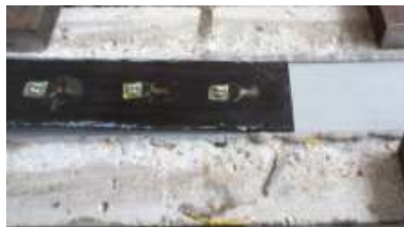
Figure 3-15 Plate-adhesive failure due to improper surface treatment
