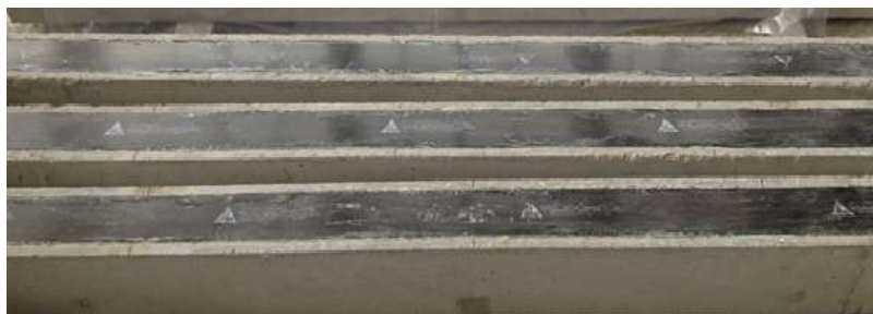
Figure 4-3 Bottom view of FRP-strengthened RC beams
