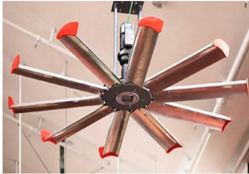
Figure 3.8 High volume low speed fan
