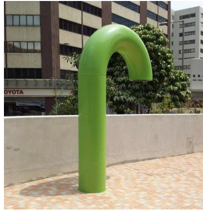
Figure 3.5 Earth cooling tube
