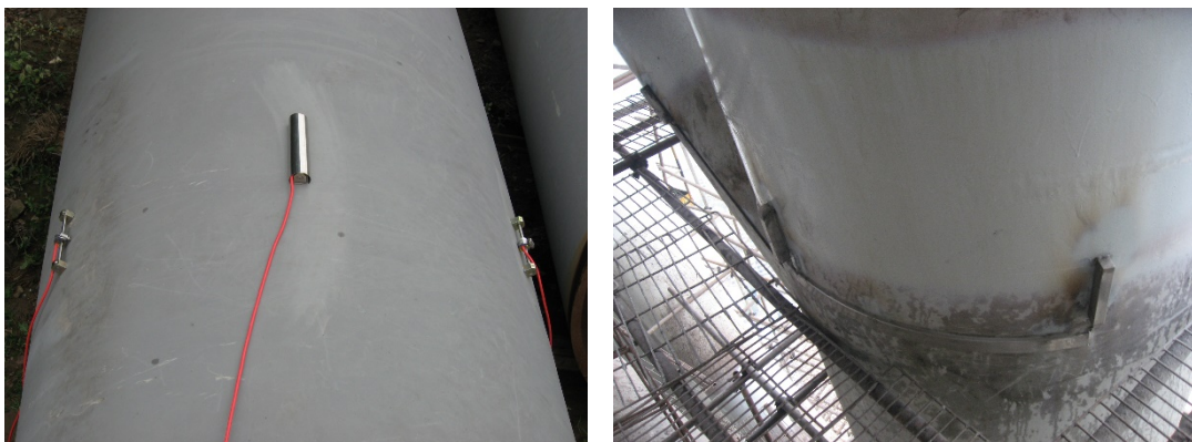
(a) Attached strain gauges
