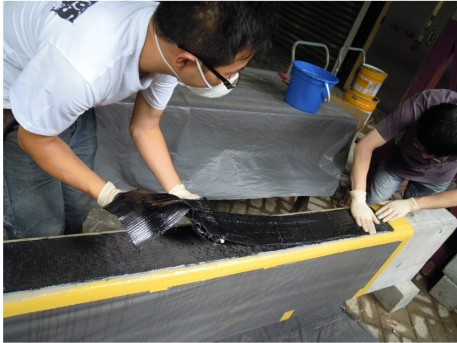
Figure A3.1.7 Application of successive layers of fibre sheets
