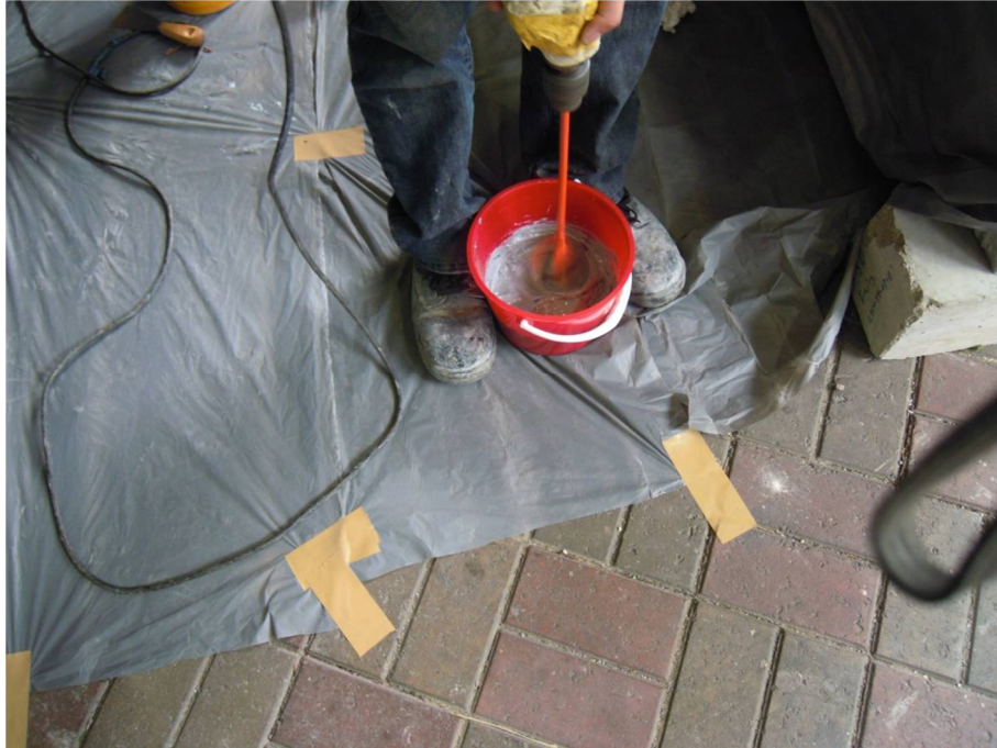
Figure A3.1.3 Mixing of primer or resin
