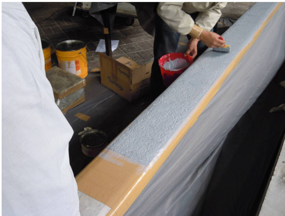
Figure A3.1.4 Application of primer
