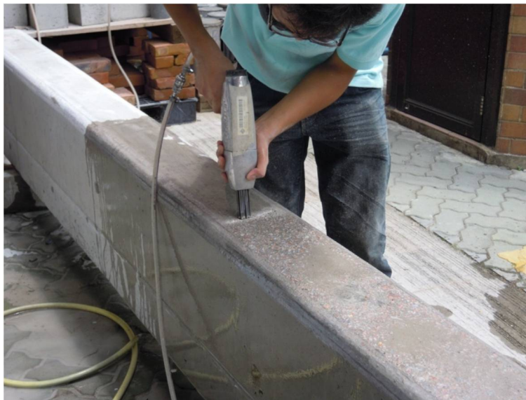
Figure A3.1.2 Profiling the concrete surface with a jet gun
