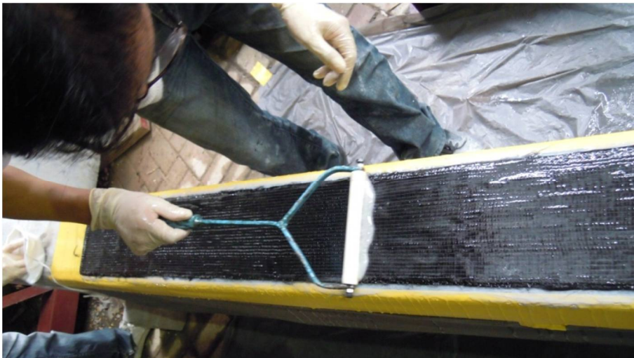
Figure A3.1.6 Slowly moving the roller to saturate the fibre sheet fully and force out excessive resin and trapped air
