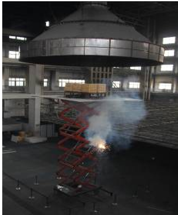
Figure 4.14 Overall situation of W5
