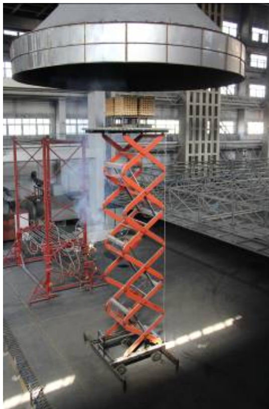
Figure 4.10 Overall situation of W3
