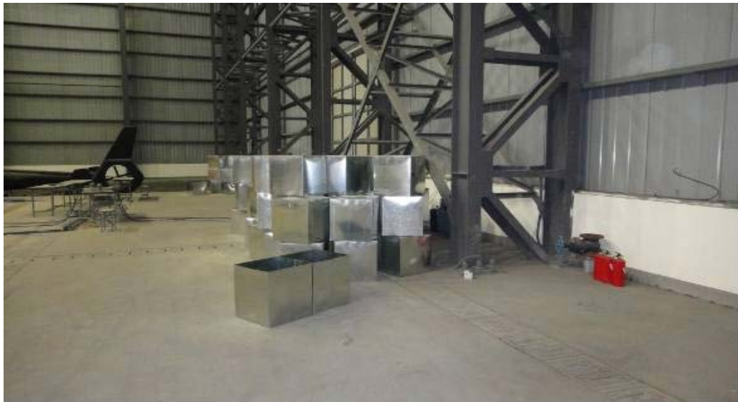
Figure 5.13 Water catchment box
