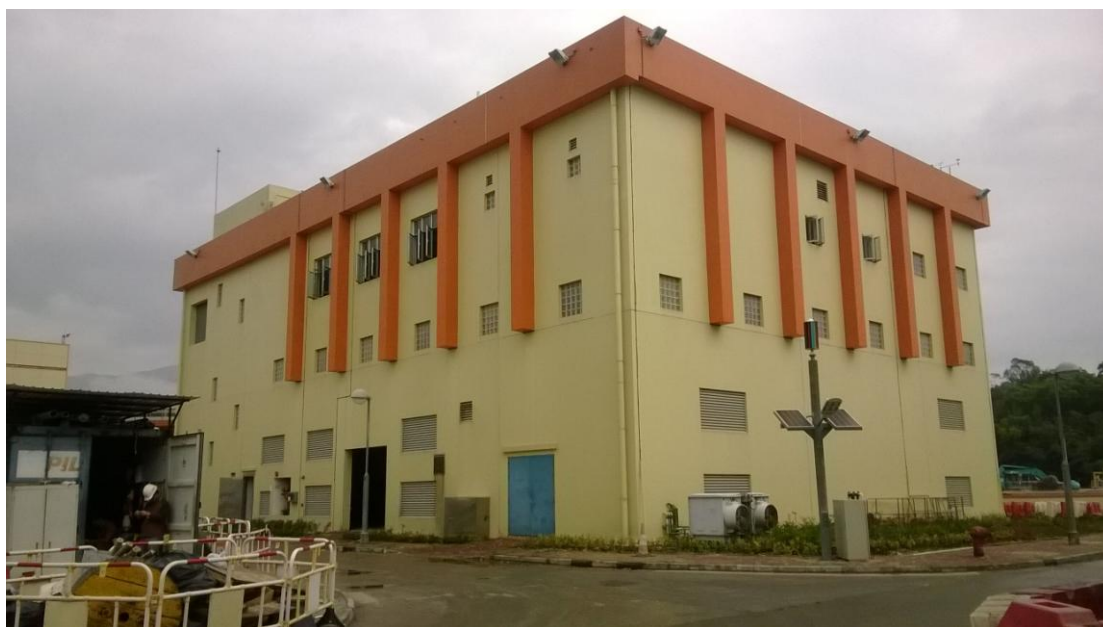
Figure 3. 9 The centrifugal facilities house in Tai Po Sewage Treatment Works
