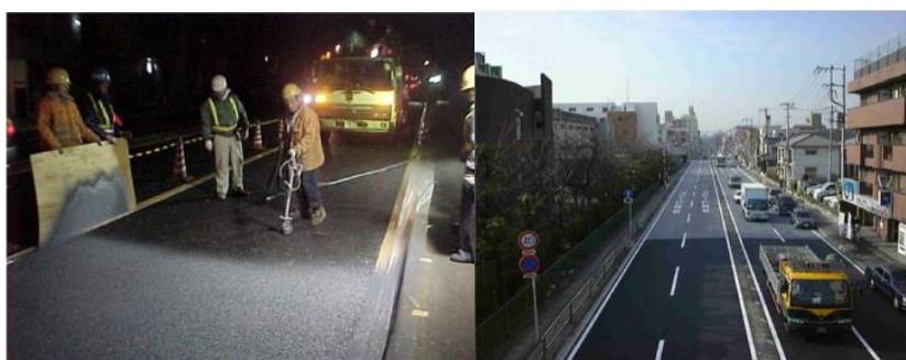
Figure 2.18 Application of TiO<sub>2</sub> photocatalytic materials on roadway for pollution reduction
