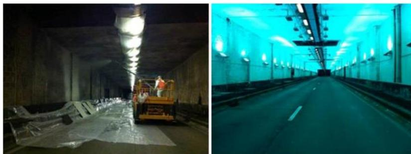
Figure 2.19 Application of the photocatalytic product and installation of the UV lamps in the Leopold II tunnel in Brussels (Boonen and Beeldens, 2014)
