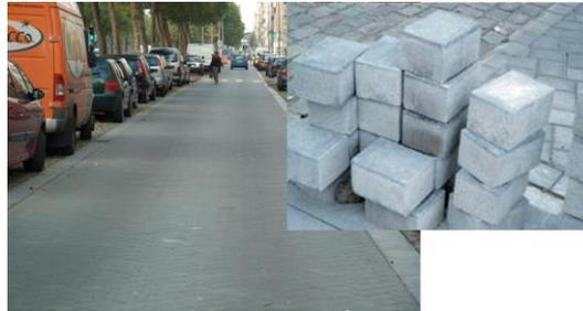
Figure 2.17 Separate parking lanes with photocatalytic pavement blocks at the Leien – Antwerp, Belgium (Boonen and Beeldens, 2014)
