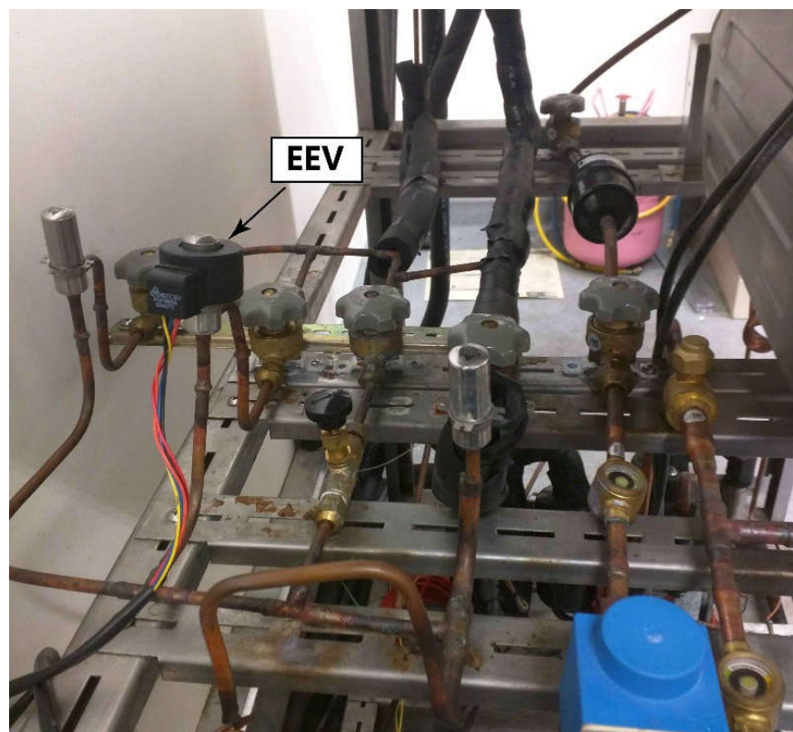
Photo 6 The EEV in the DX refrigeration plant
