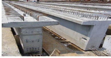
Precast Tie Beam
