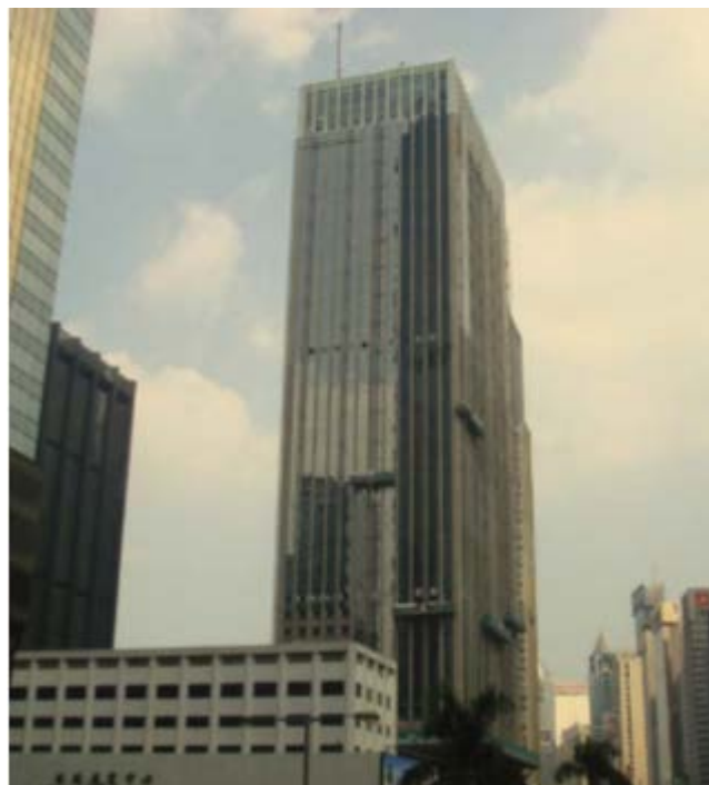
Figure 38 China Resource Building GRD project
