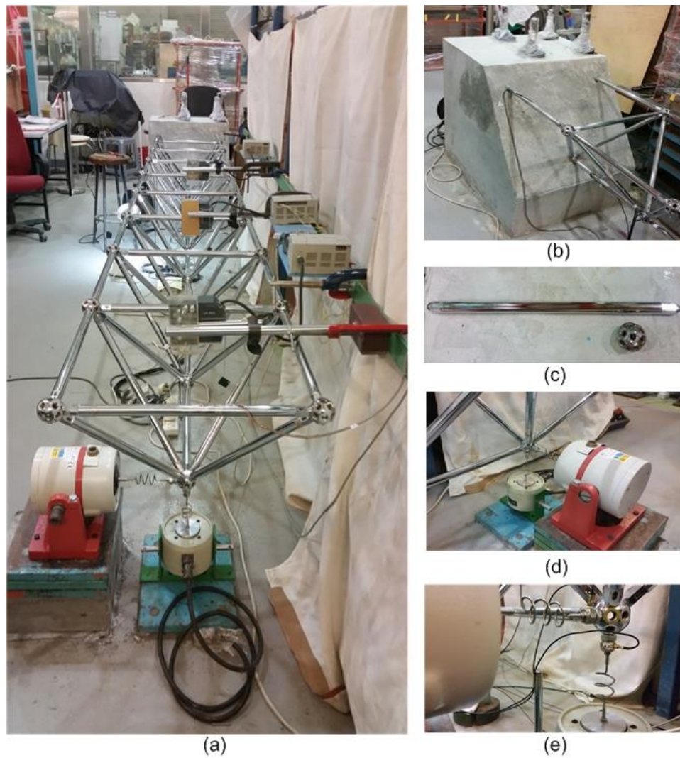
Fig. 6.1 The physical model of the nine-bay frame structure and experimental setup: (a) The nine-bay frame installed with two exciters; (b) The rigid concrete support; (c) The alloy steel tube and Meroform ball; (d) Two exciters LDS V406 M4-CE & JZK- 5; (e) The springs and B & K force transducers.
