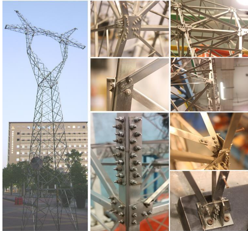
Fig. 7.1 The straight-line type 5A-ZB2 HVPT tower and its bolted joints
