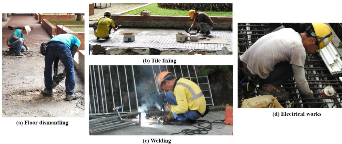
Figure 4.10 Other construction tasks requiring squatting postures
