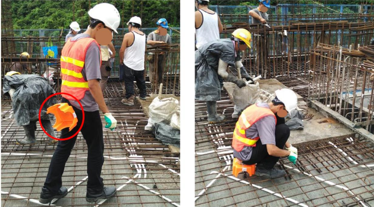
Figure 4.1 Attachment of a stool to the trousers using self-adhesive Velcro straps
