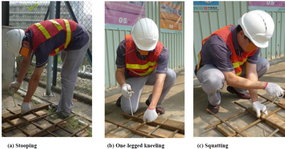
Figure 3.1 Three postures of rebar tying
